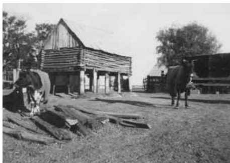
Shed with cows, and the collapsed shed below in 2008.
