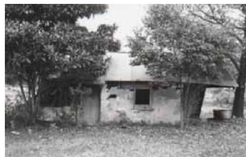
The schoolhouse in disrepair in 2008 and below in the demolition period in 2009.
